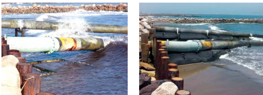
FIGURE 9 Before-and-after comparison for pipes 6 and 7
