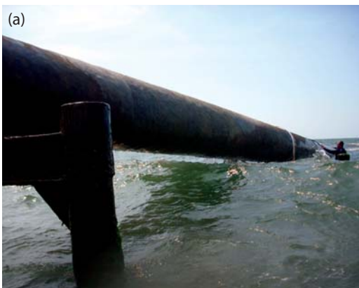
Geotextile tubes filled with sand work as foundations and support beds for oil pipes at the Dos Bocas facilities for Petroleos Mexicanos. Below: (a)—At some locations, gaps between the sea floor and pipe were more than 2m. (b) & (c)—The geotextile tube foundations were designed to fill the gaps for each pipe. See also Figure 3, page 31.
