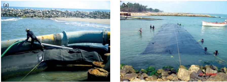
FIGURE 6 Filling GT tasks: (a) pipe support elements and (b) breakwater
